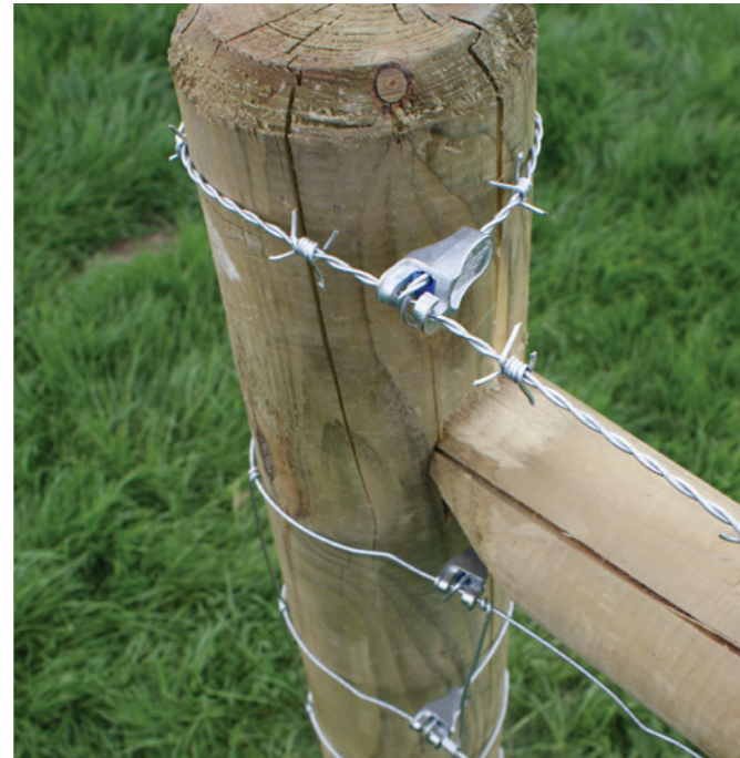
T-Clip 2 - Used to terminate barbed wire.
