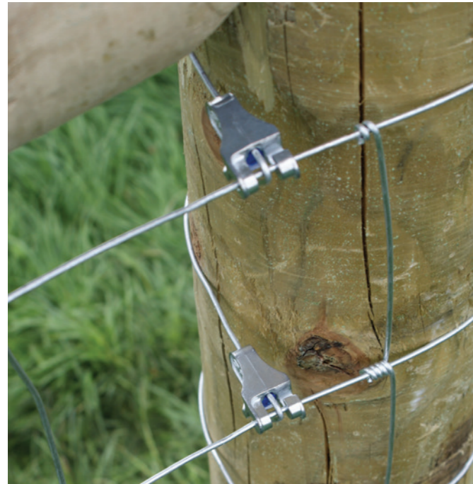
T-Clip 1 - Installed on a stock fence.
